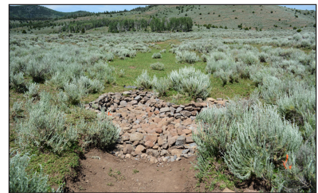
Here this structure is done. It will stop the erosion moving up valley and catch sediment and help fill in the gully. Several of these were built around this valley bottom.
