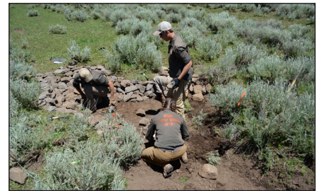
Hand built rock structures are commonly used to control erosion in meadows. They are low cost-high reward conservation practice.
